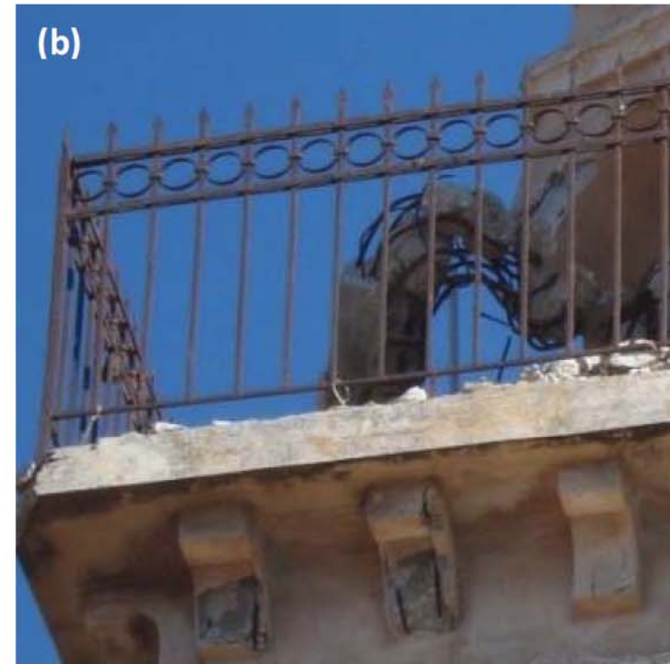
Figure 11.8.13. (a) Collapse of RC belfry top due to column failure ( 38^{\circ}14'32.25''\text{N} , 20^{\circ}28'26.40''\text{E} ); (b) Detail of deformed rebars.
