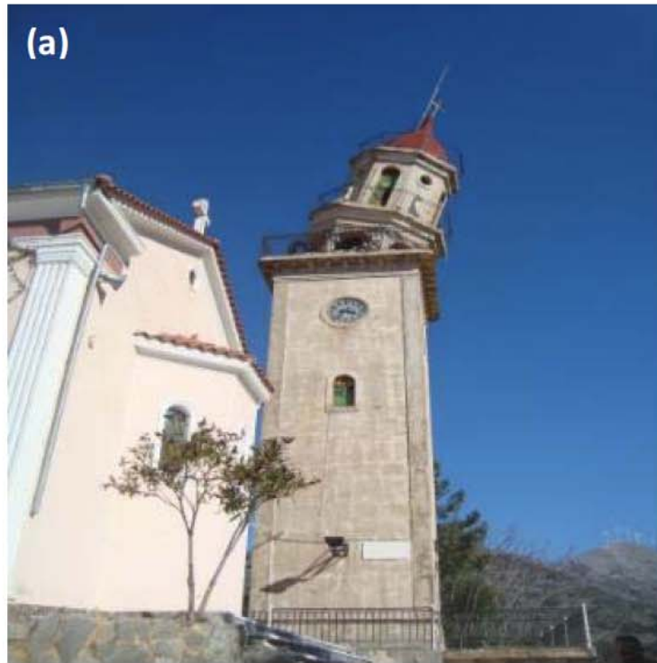
Figure 11.8.13. (a) Collapse of RC belfry top due to column failure ( 38^{\circ}14'32.25''\text{N} , 20^{\circ}28'26.40''\text{E} ); (b) Detail of deformed rebars.
